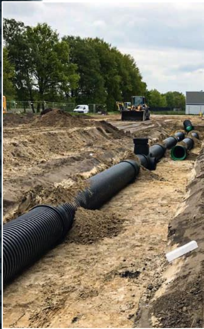
AQUATUB-Rw DN 600 in combination with the MULTI-inspect MONO chamber system
